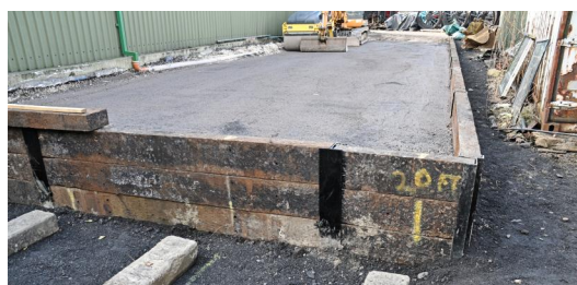
The base for the new work area.
