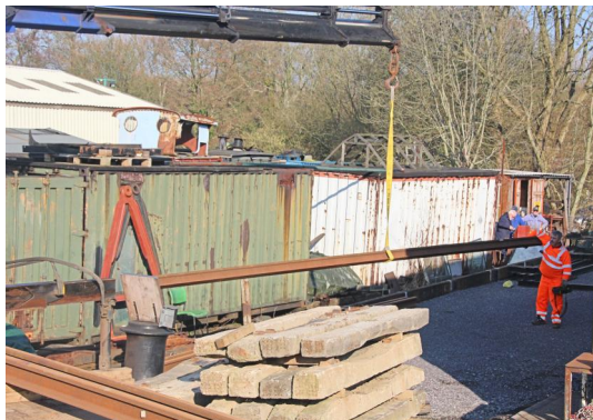
Recycled flat bottom rail being offloaded
