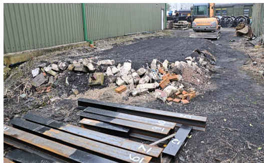
Site at ready for start of Civil Work
